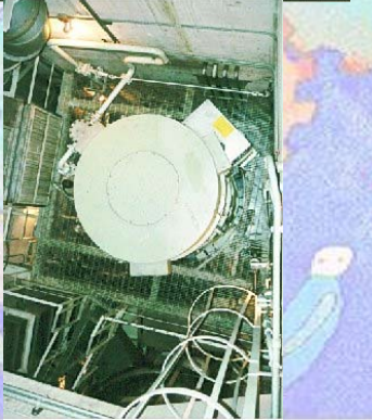
Assembly of a reactor coolant pump (Photograph by courtesy of Klein, Schanzlin und Becker)
